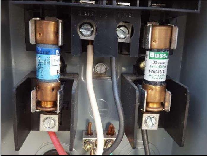
30-amp fuses installed
